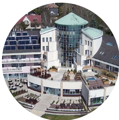
Telekom Hotel Balatonkenese
